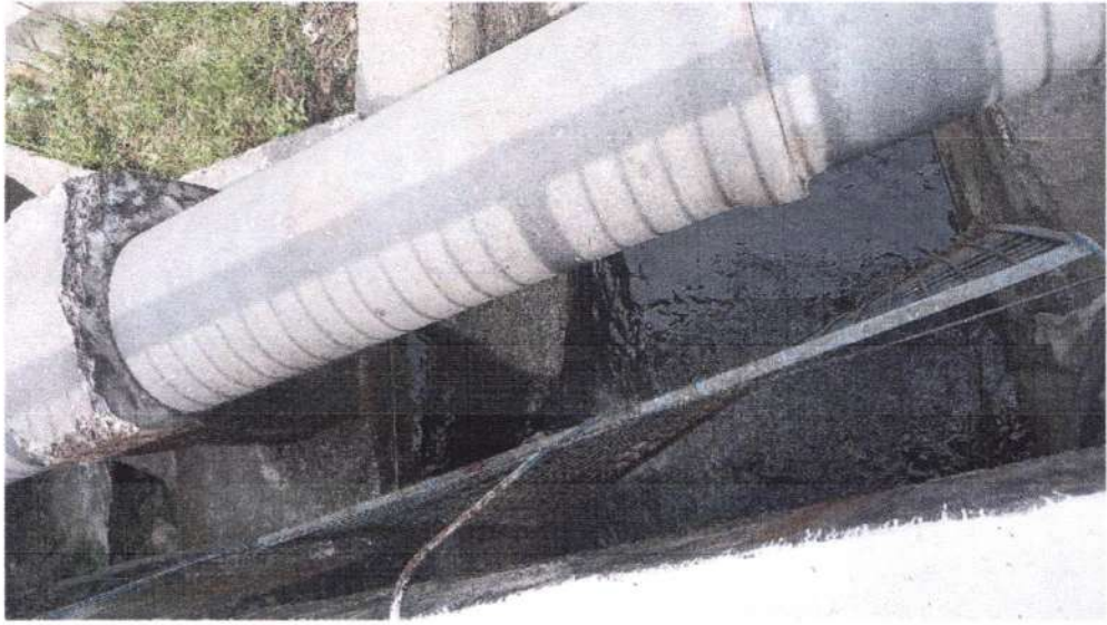
Shahid nagar drain VIP road
